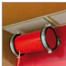
Fire extinguishing generator
